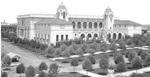
写真10: Southern California Counties Building
